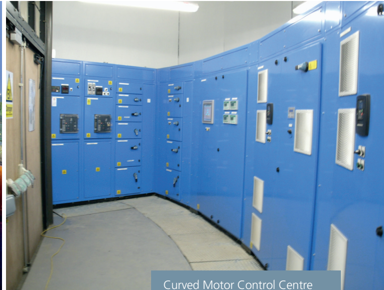
Curved Motor Control Centre (MCC) designed to maximise space
